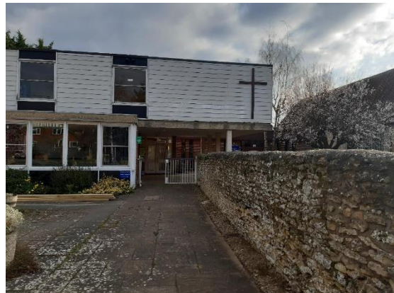
Pedestrian access from the road,
