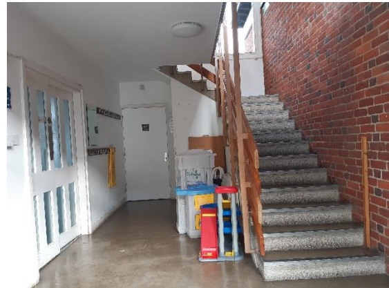
Stairs to upper room, toilet entrance
